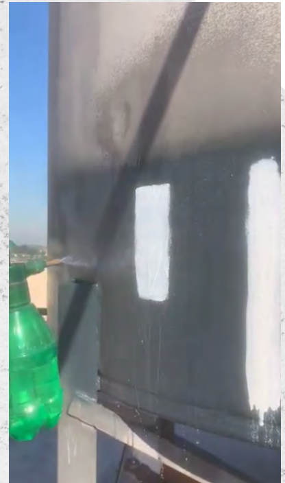
H2Poxy can be applied to wet substrates. Here, water is sprayed onto newly applied H2Poxy-A that was rolled onto vertical wet metal.
