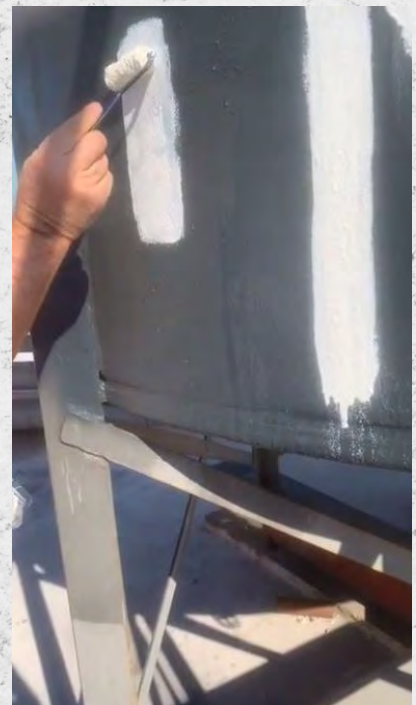
H2Poxy is extremely water resistant even when in an uncured state. Applied to a vertical surface, it will not drip or fail to adhere.
