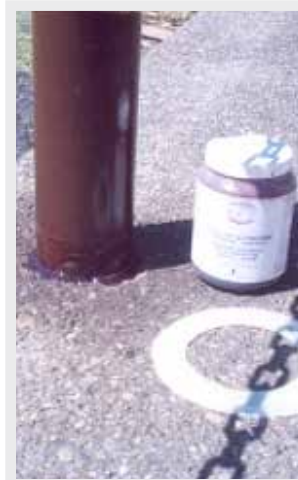
Ready for fiberglass ring.
